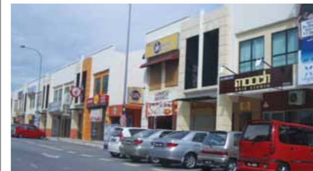
Fortune Square 2 @ Kepong, KL
