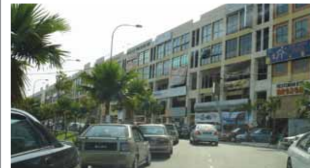
Fortune Square @ Kepong, KL
